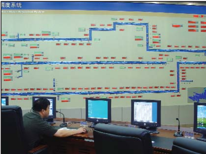
An operator accesses the Yellow River's plant intelligence and supervisory control system through the Industrial Application Server Integrated Development Environment.
